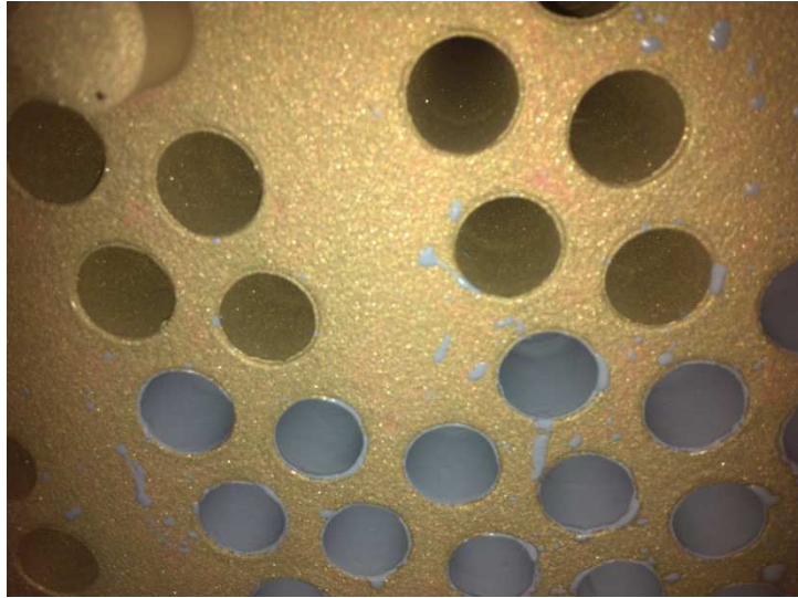
Tube coating in progress.
