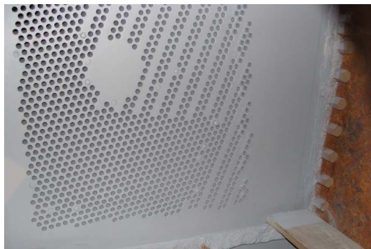
Above are pictures of the outlet tubesheet with a single coat of Phenolic Epoxy applied to tie in the tube coating with the tubesheet.
