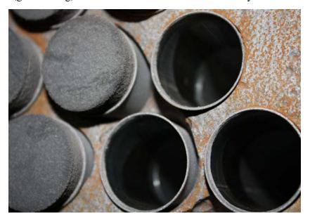
Tube-sheet after grit blasting. Note how even the small tube to tube-sheet crevasse is blasted clean.
