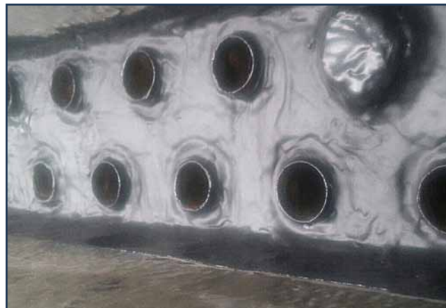
Tube Plate After Coating
