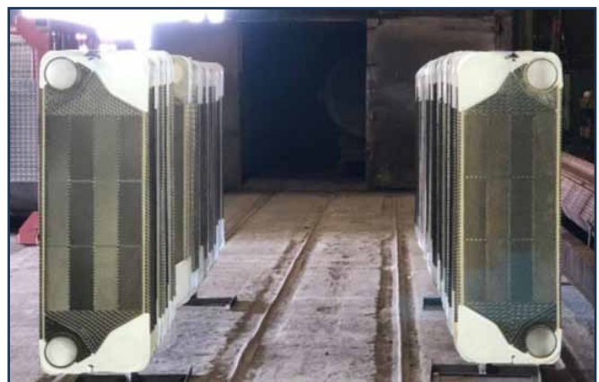
Plates with gasket areas properly masked off prior to coating.
