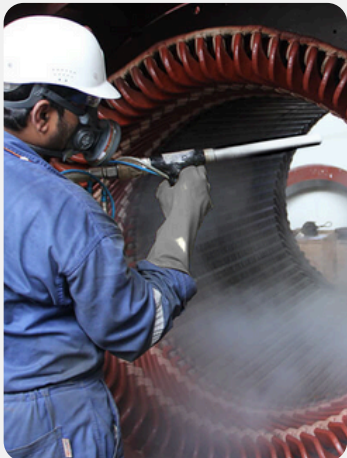
Steam Turbine Grit Blasting
