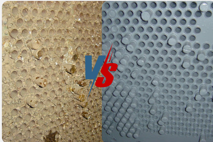
Before & After Condenser Tube ID & Tubesheet Coating
